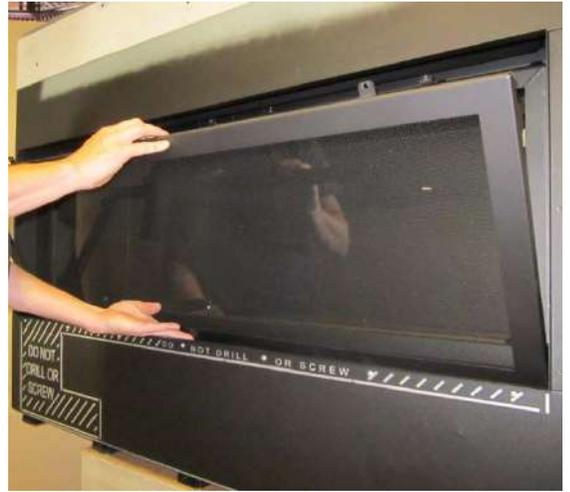
3. Use the glass tool to unlatch the glass frame. Remove the glass frame. The glass frame is held in place with four tabs inserted into four slots at the bottom of the firebox opening.
